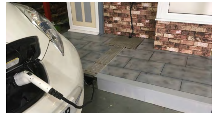
Figure 18 Example of a gully & cable protector
